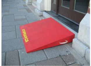
Figure 21 - Customized portable ramps are a simple method to improve accessibility
