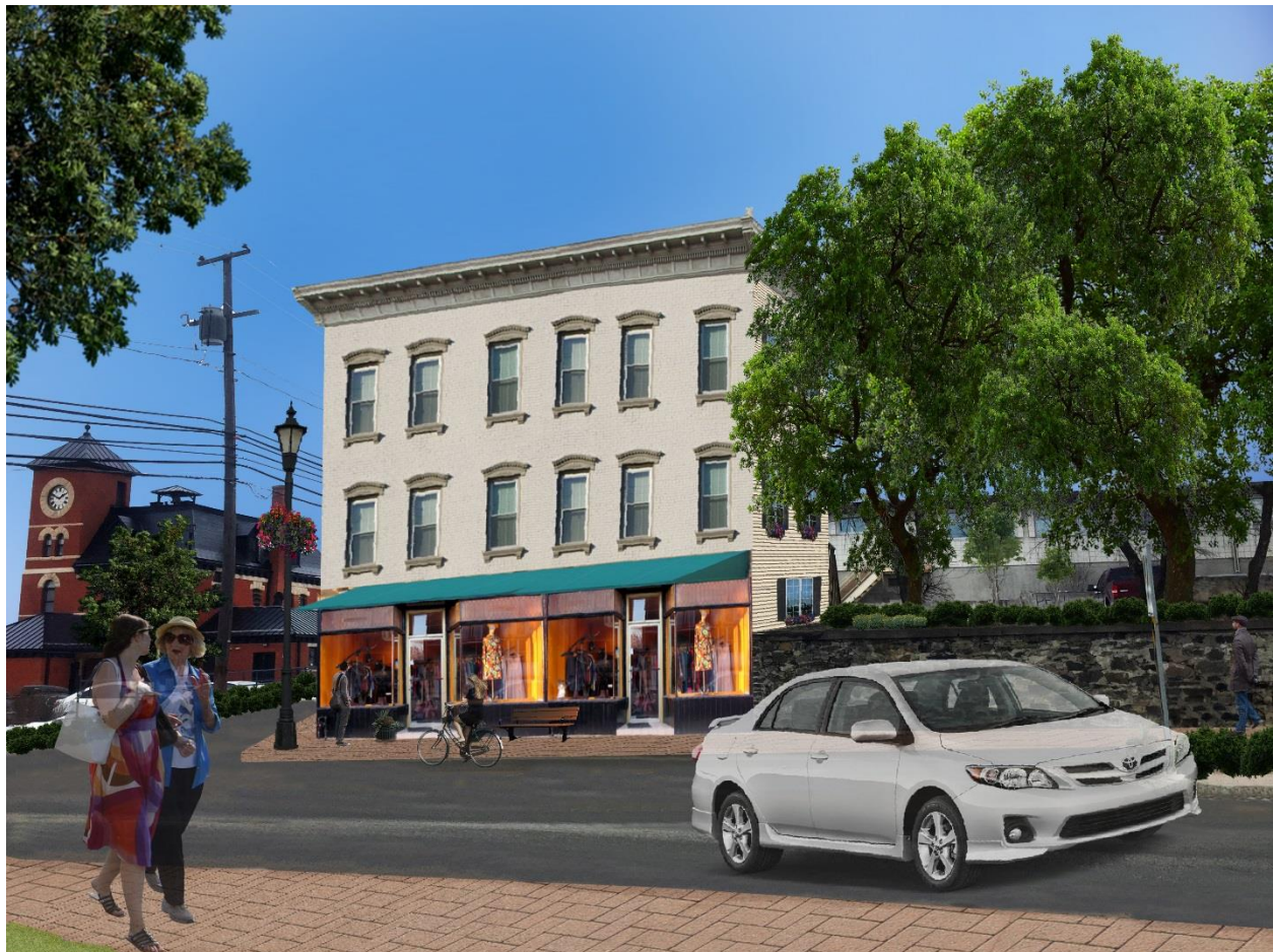
Figure 3 - McClellan Avenue and Hennepin Lane now (top image) and after improvements funded in part by CIP grants (below).
